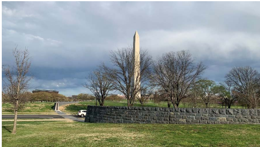
Figure 6-7. New Flood Wall on the National Mall – 17th St NW
